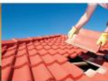
Roof Replacement 67% ROI
